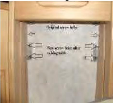
Now install the 4 wall screws where the wood braces are now located, the removed screws are self tapping. Be careful not to tighten the screws to tight as they will strip.
